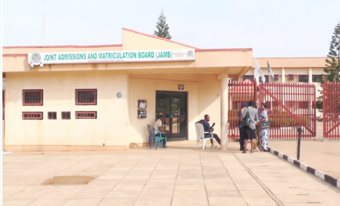
OLD GATE HOUSE AT THE HEADQUARTERS
