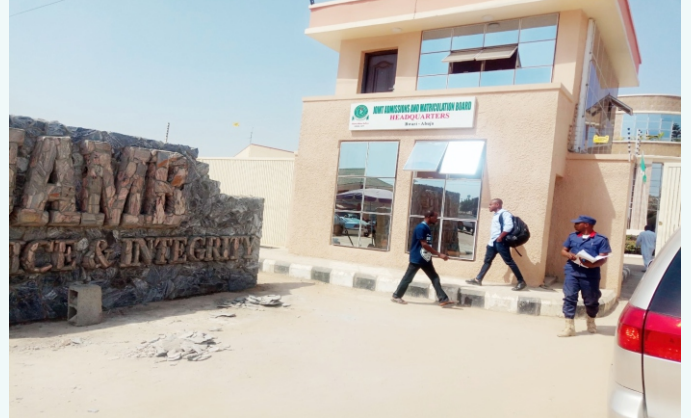
NEW GATE HOUSE AT THE HEADQUARTERS
