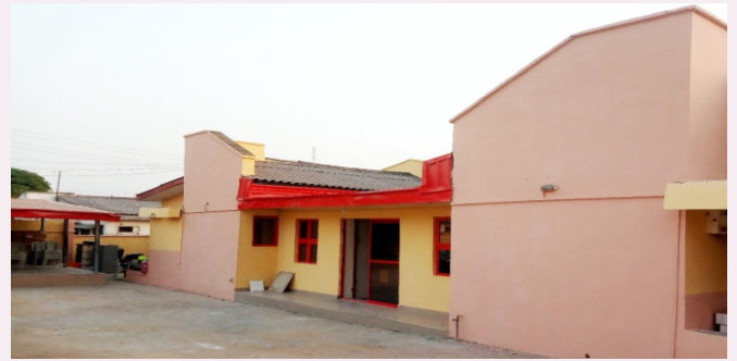
NEW KOGI OFFICE
