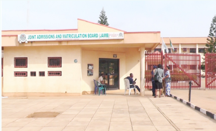
OLD GATE HOUSE AT THE HEADQUARTERS
