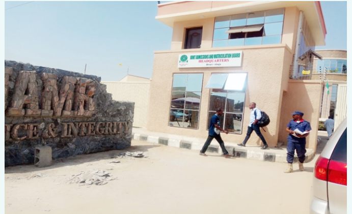
NEW GATE HOUSE AT THE HEADQUARTERS
